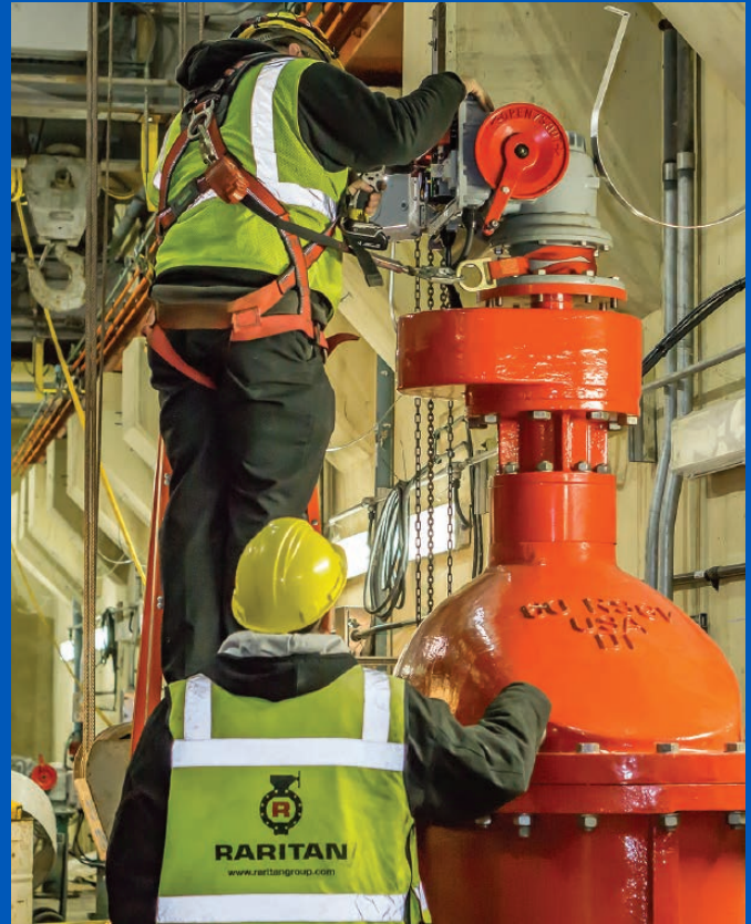
RVA technicians commission 60" gate valve
