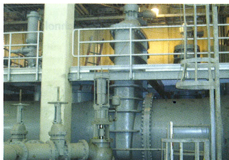
72" Resilient Seated Gate Valve – Largest Resilient Seated Gate Valve in the USA
